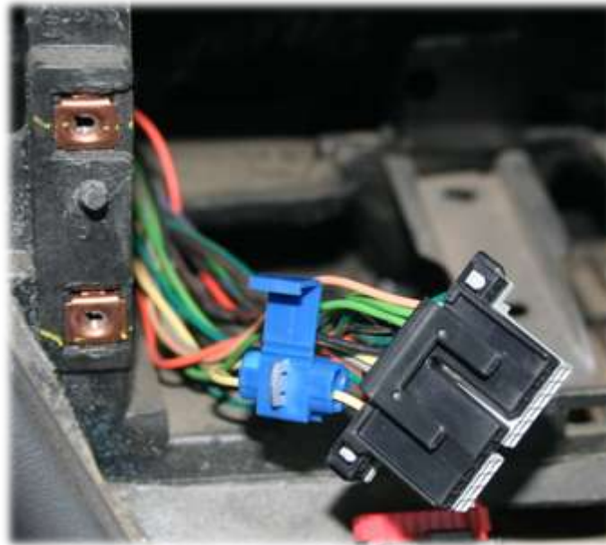
Image 6: Scotchlok Connector Being Installed
